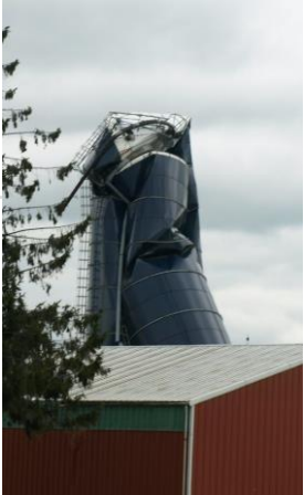
"Fail Silo" by thetorpedodog is licensed under CC BY-SA 2.0
